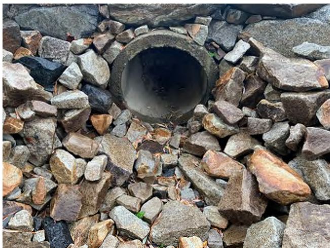
64 Gundalow - 1 (Drainage Course)
