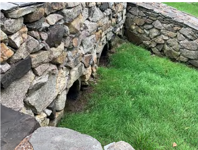
4 Brickyard Circle - 1 (Drainage Course)
