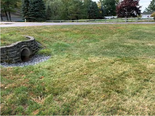
29 Gundalow - 1 (Drainage Area)
