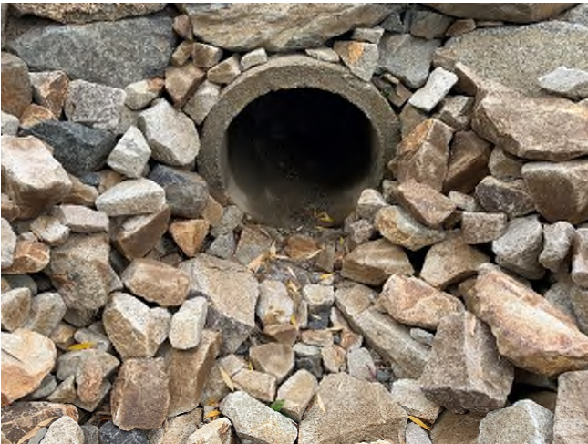
64 Gundalow - 1 (Drainage Course)
