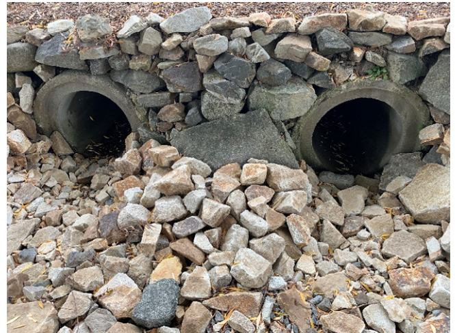
64 Gundalow - 2 (Drainage Course)
