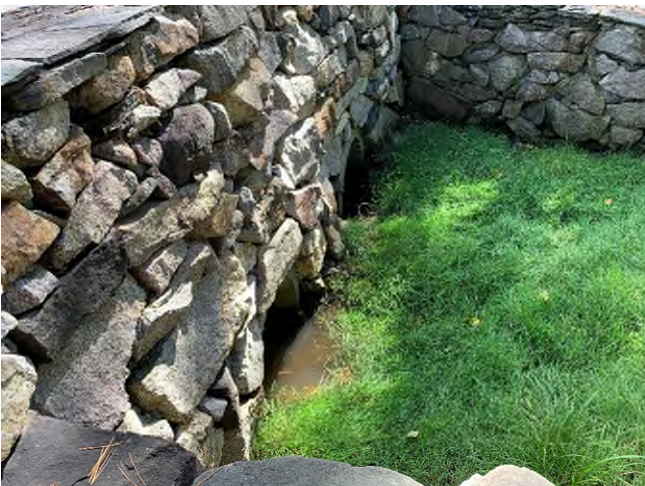
4 Brickyard Circle - 1 (Drainage Course)
