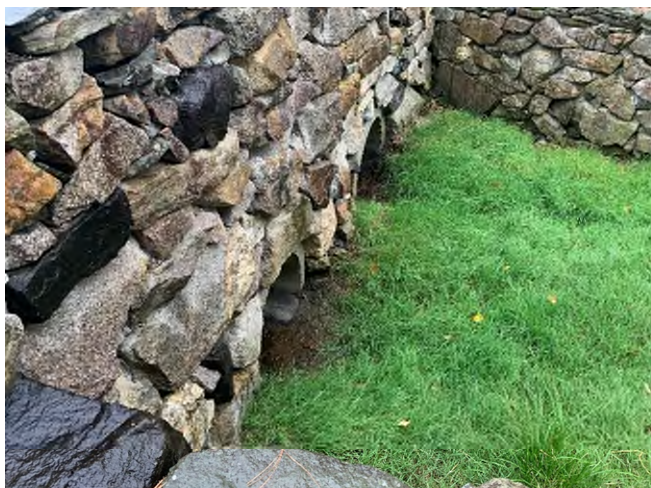
4 Brickyard Circle - 1 (Drainage Course)
