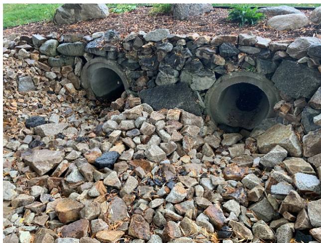
64 Gundalow - 2 (Drainage Course)
