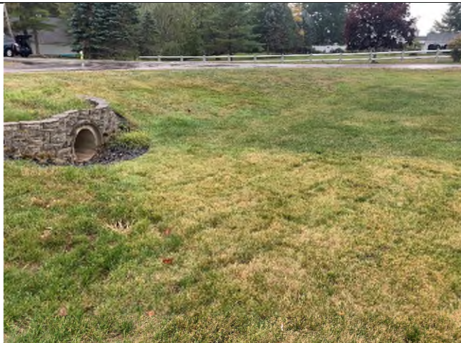
29 Gundalow - 1 (Drainage Area)
