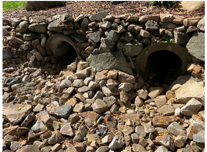
64 Gundalow - 2 (Drainage Course)
