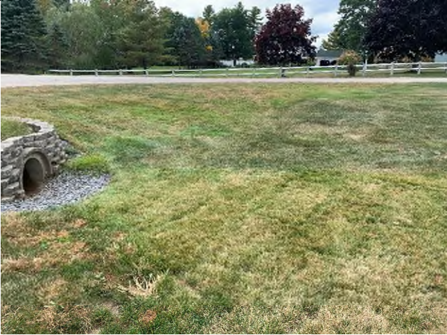
29 Gundalow - 1 (Drainage Area)
