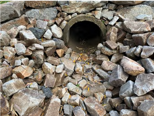
64 Gundalow - 1 (Drainage Course)
